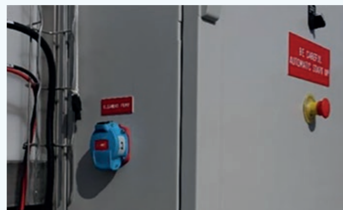
Electric plug for the cleaning pump, included in the OSMOSUN® cabinet
